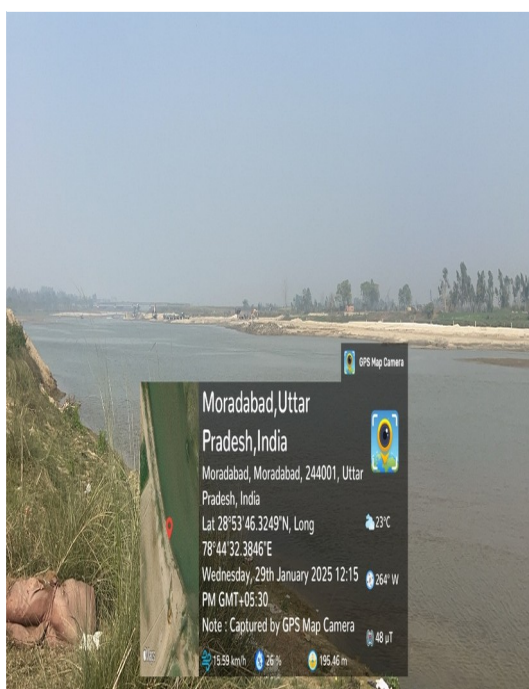
River Bank Inspection
