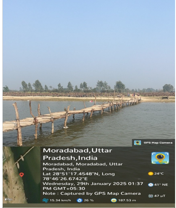
Inspection of Water Body
