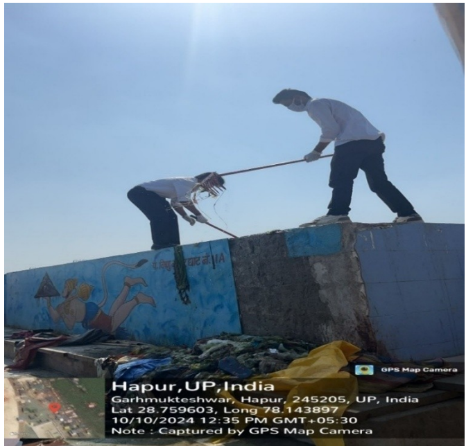
Work at Site
