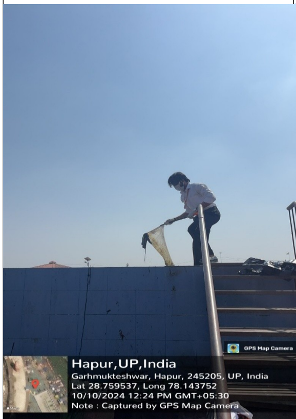
Work at Site
