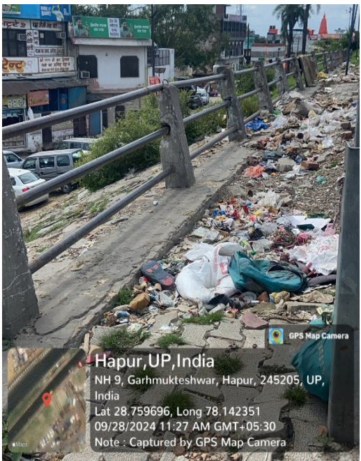
Road Side Garbage on Bridge
