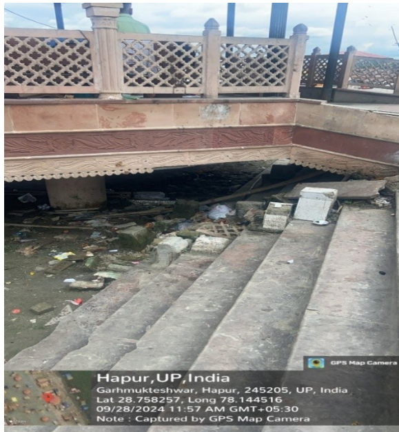
Inspection of Staircase Area
